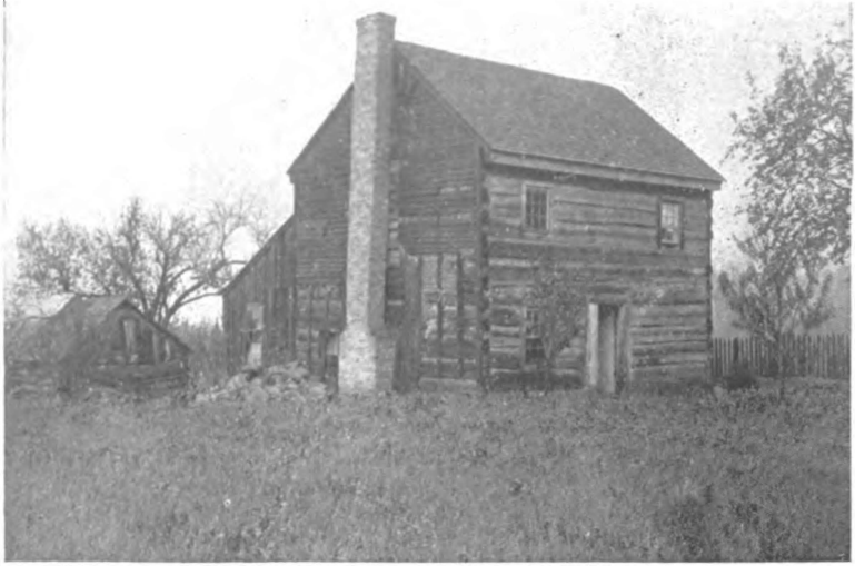
House Built By William Ewing, at Ewington, Ohio, 1812.
